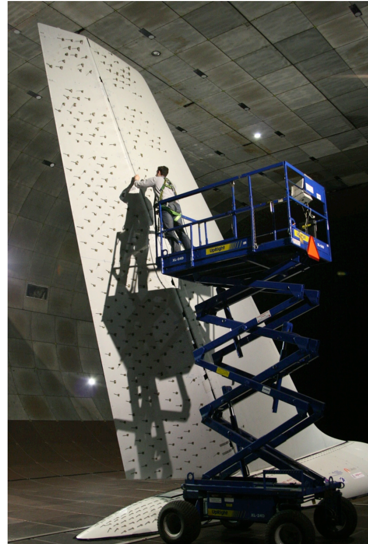
757 AFC Enhanced Vertical Tail installed in NFAC End of day tuft maintenance
